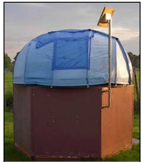
Three years of UV radiation and wind storms takes its toll on the tarp dome.
